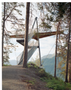
17 Viewing platform / Corinna Menn Architektin ETH/SIA / Photo: Franz Rindlisbacher
