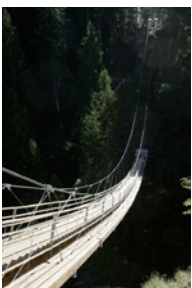
16 Traversiner footbridge / Conzett, Bronzini, Gartmann AG / Photo: Wilfried Dechau
