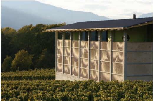
I_ Exterior view of the Gantenbein Winery © Ralph Feiner
