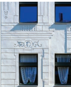
XXX_Façade Refurbishment Berlin-Schöneberg: Detail view © Michael Heinrich
